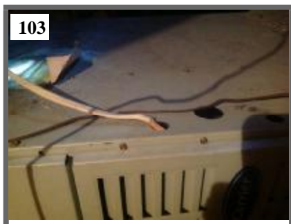
Unprotected wire going into furnace
