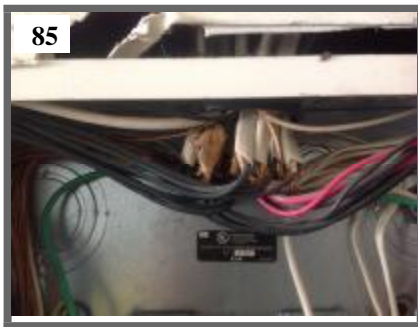
Conductor wires entering one knockout
