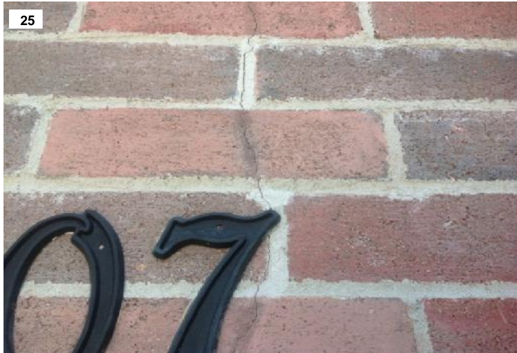
Crack in brick veneer located above garage
