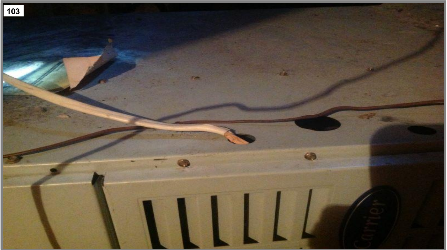
Unprotected wire going into furnace
