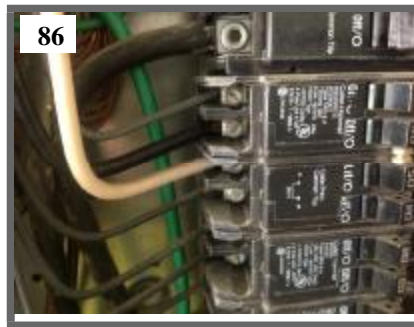
Neutral wire used as hot wire
