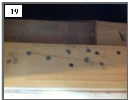
improper attachment of pull down stairs
