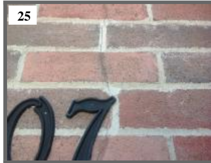
Crack in brick veneer located above garage
