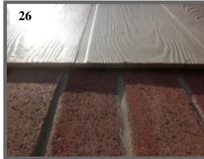
siding to brick needs caulking
