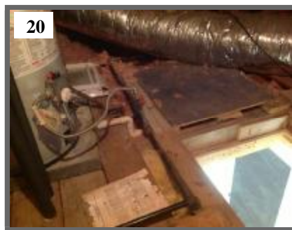
improper working platform in front of water heater
